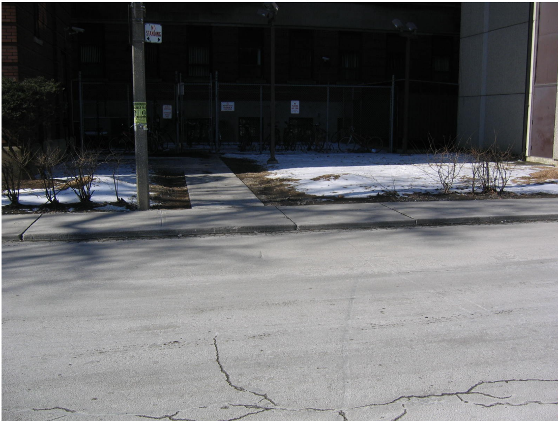
30 Bond Street, St. Michael's Hospital February 12, 2010
