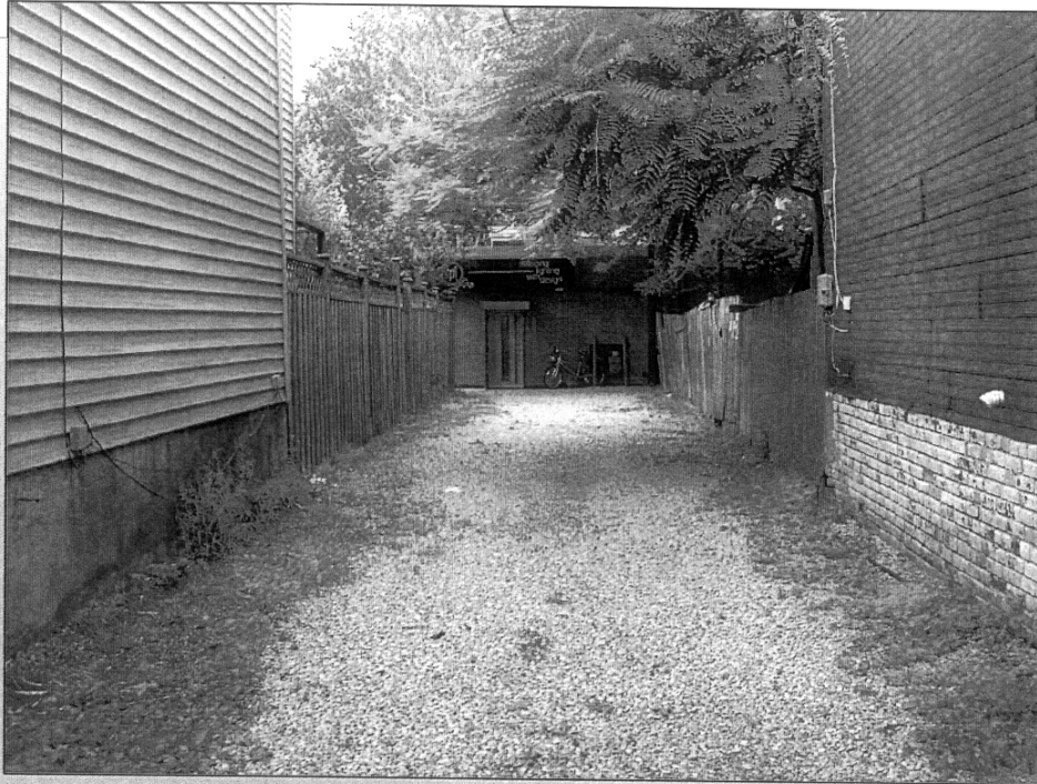
WEST ELEVATION OF BUILDING
