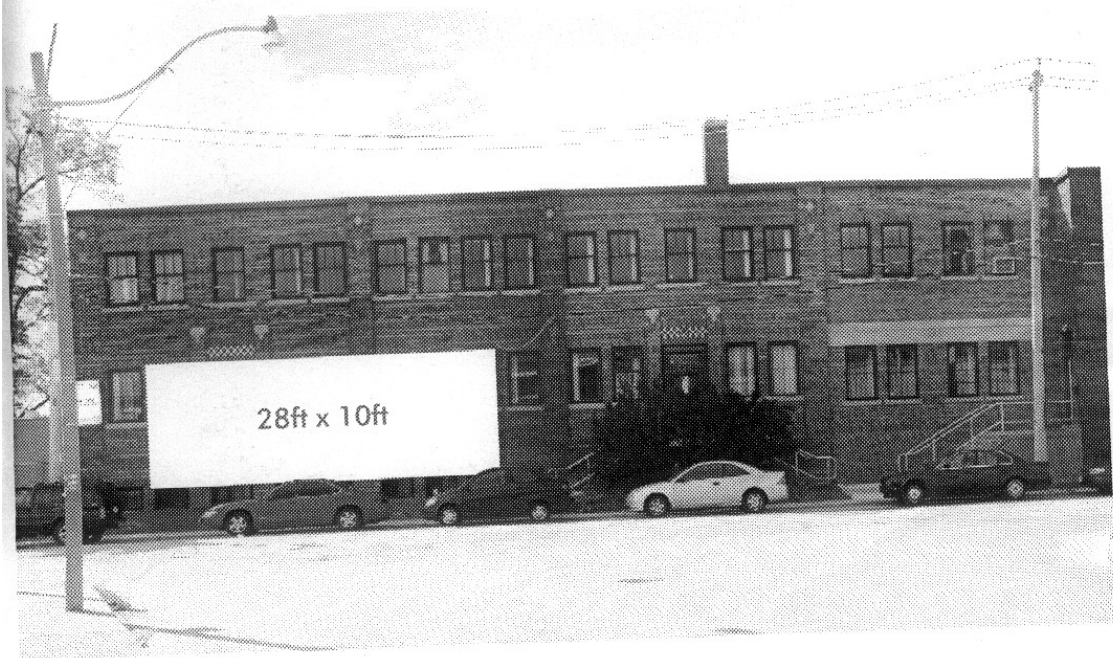
view looking south from St. Lawrence St.
