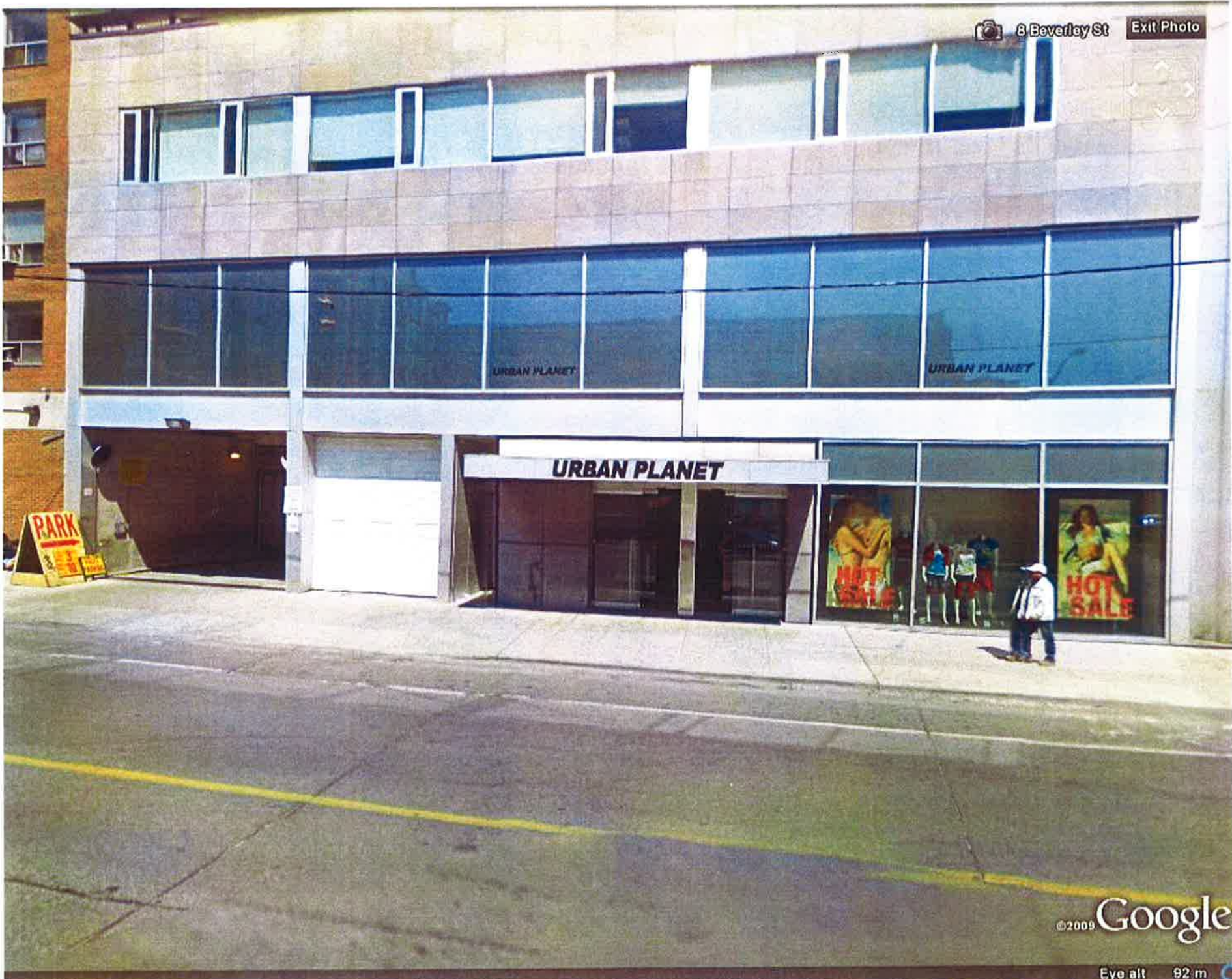
Existing conditions. Signs to be removed & replaced with new
