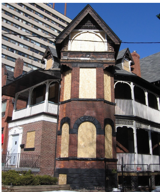
Above: detail, southwest bay
