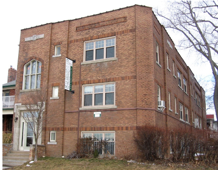
Hubbard Court Apartments, showing the principal (south) façade (left) and east elevation (right)
