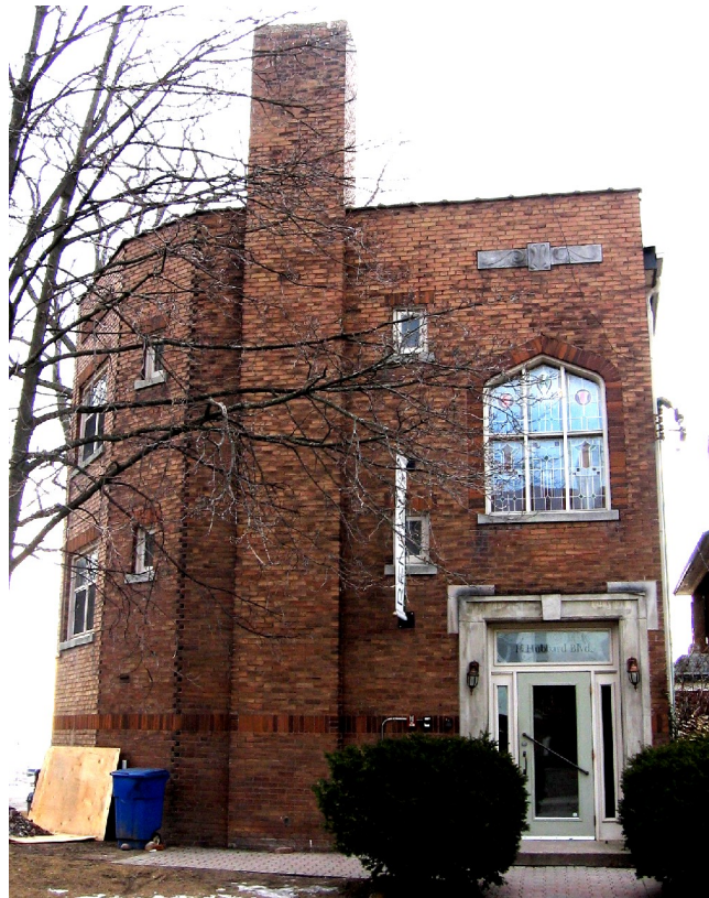
Rear (north) wall with north entrance (right) and bevelled northeast corner (left)
