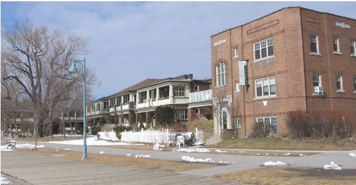
View of the subject properties on Wineva Avenue (left) and Hubbard Boulevard (right), with the Boardwalk in the foreground.
