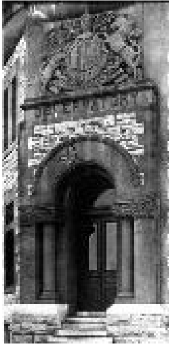
Detail of the Royal Observatory, Ottawa, which inspired the design of the Dominion Meteorological Building in Toronto (City of Toronto Archives, Fonds 1244, Item 9173)
