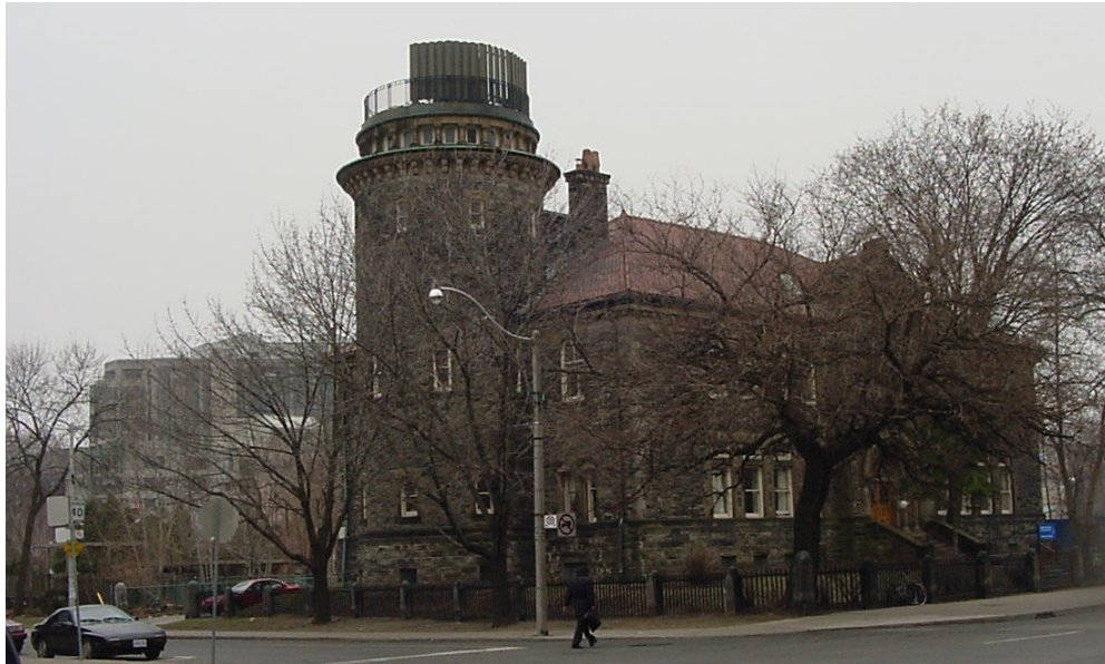
Contextual view of the Dominion Meteorological Building on the southwest corner of Bloor Street West and Devonshire Place
