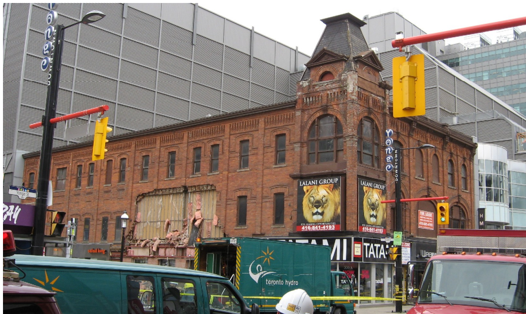
Photograph taken on April 16, 2010, showing the partial collapse of the north façade (left) on Gould Street
