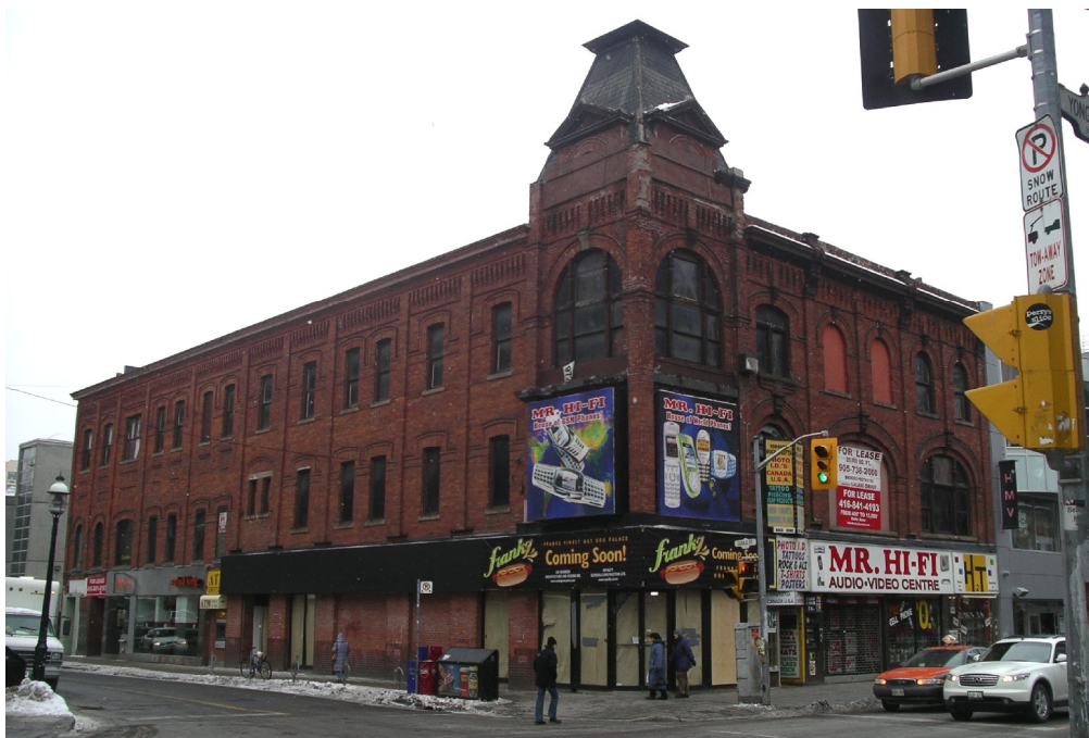
335 Yonge Street, showing the west (right) and north (left) facades
