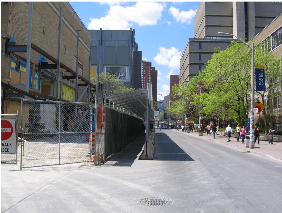
122 Bond Street – Gould Street flank looking west towards Yonge Street – May 3, 2010
