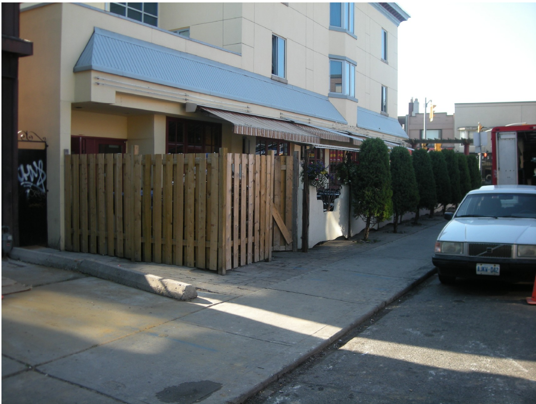
390 Danforth Ave – Garbage bin storage enclosure on Chester Avenue flank, Danforth Avenue to the right, May 25, 2010
