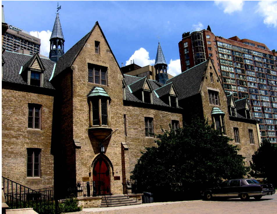
South façade of the Cloverhill Wing, July 2010
