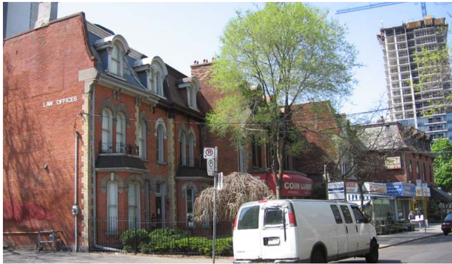
William McBean Houses at 25-35 Howard Street, with #35 on the left. The William McBean Stores at 21-23 Howard Street are shown on the right and on the cover of this report
