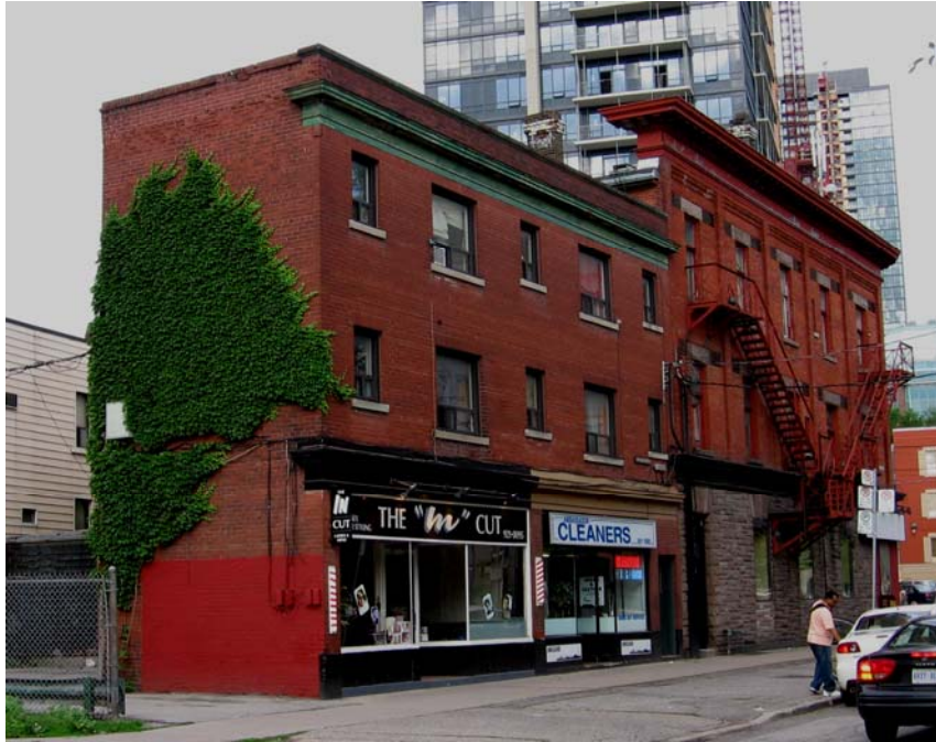
View of the north elevation on Howard Street with the rear (east) wing
