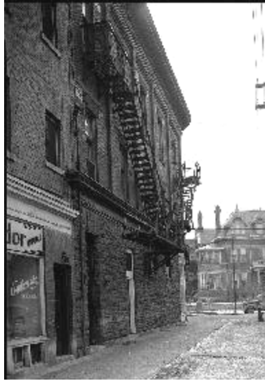
Photograph looking west on Howard Street, showing the north elevation of the Thomas Cruttenden Building (left), with the James Cooper House at 582 Sherbourne Street in the background (centre) (Source: City of Toronto Archives, Fonds 200, Item 1600, January 15, 1942)
