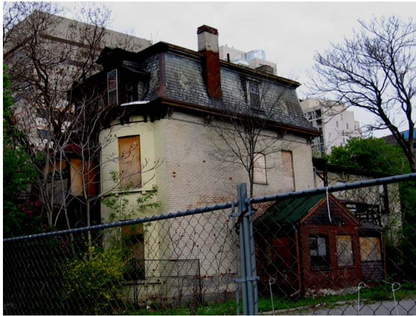
Photograph showing the south (left) and east (right) elevations of 4 Howard Street, 2010
