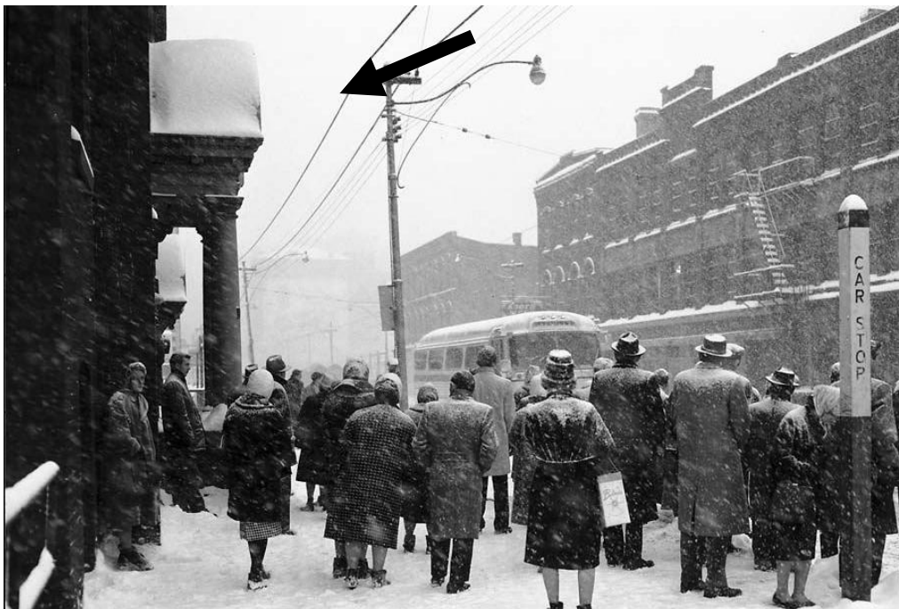
Photograph showing the portico of the Eclipse Whitewear Building (left), 1961 (Source: City of Toronto Archives, Fonds 1257, Item 25)
