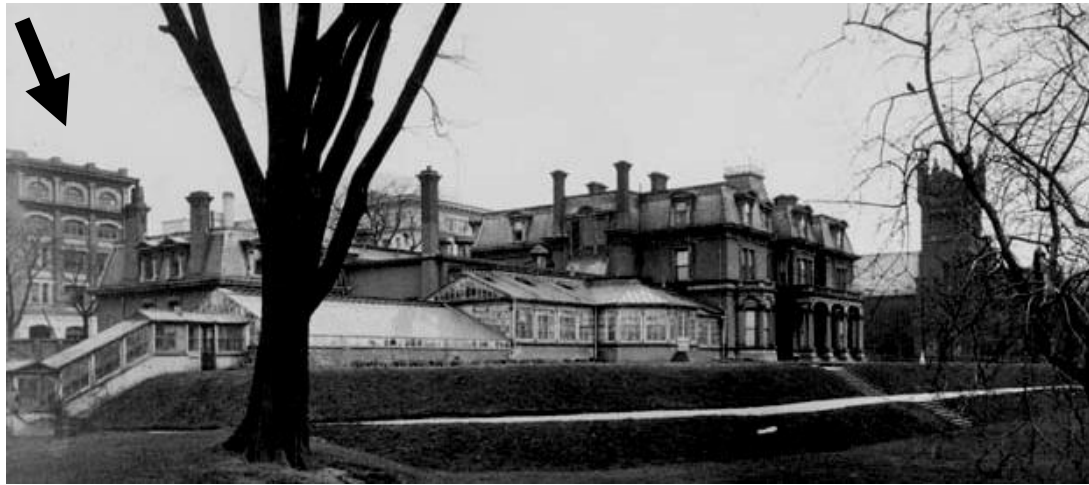
View of the Nicholls Building (left) on the north side of King Street West, opposite Government House (which fills the centre of the photograph), in 1912 (Source: Library and Archives Canada, Item 25592)
