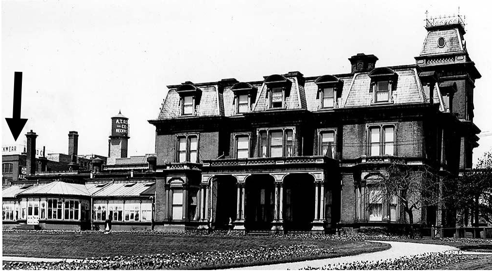
Photograph dated 1909, showing the second Reid Building (1909) in the background on the left (with Government House in the foreground) (Source: City of Toronto archives, Fonds 1244, Item 3035)
