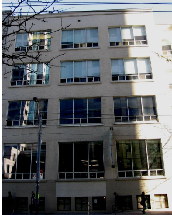
Photograph showing the south façade of the 1942 west addition to the Gillett Building
