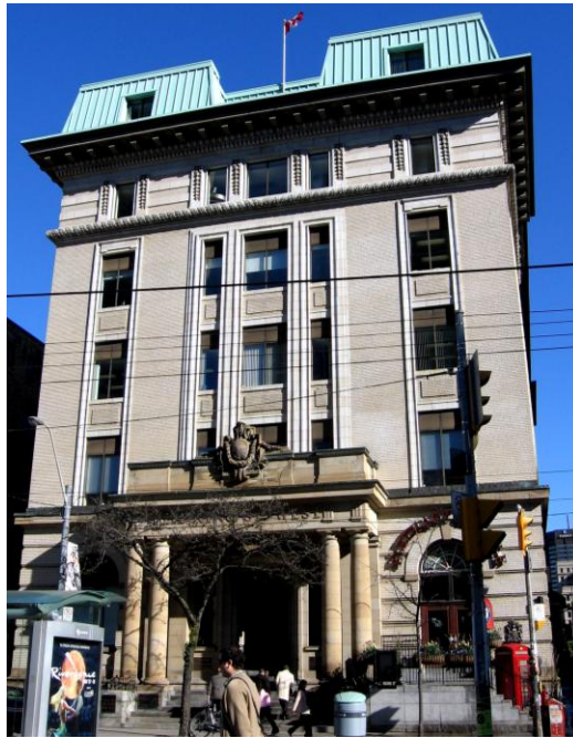
Principal (south) façade of the Union Building (the sixth floor with the mansard roof is an addition)
