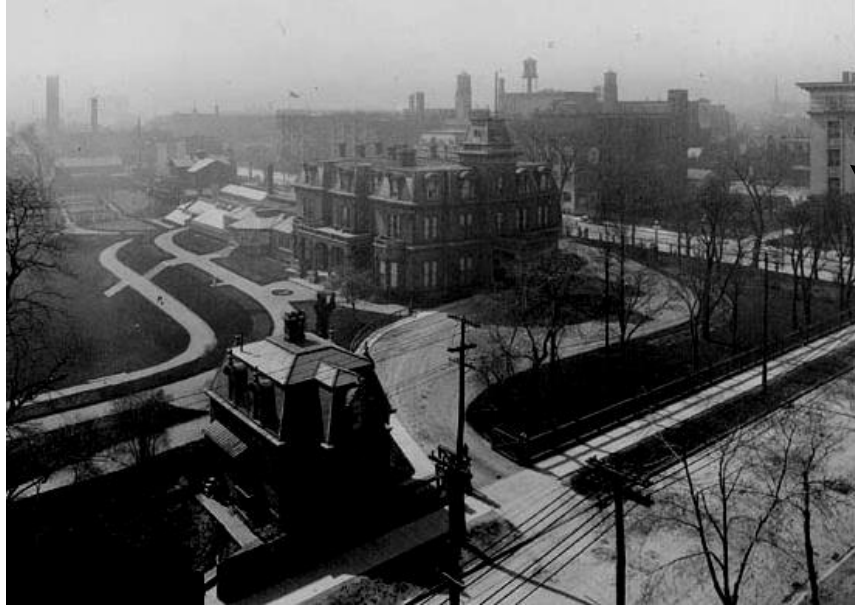
Photograph dated circa 1908 showing part of the recently constructed Union Building on the right, where it overlooked Government House on the southwest corner of King Street West and Simcoe Street (Source: Library and Archives Canada, Item 25593)
