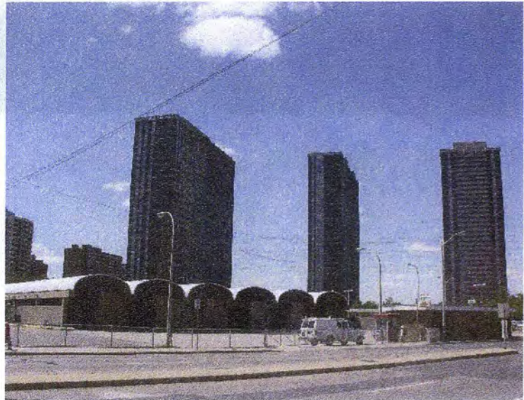
north west corner
