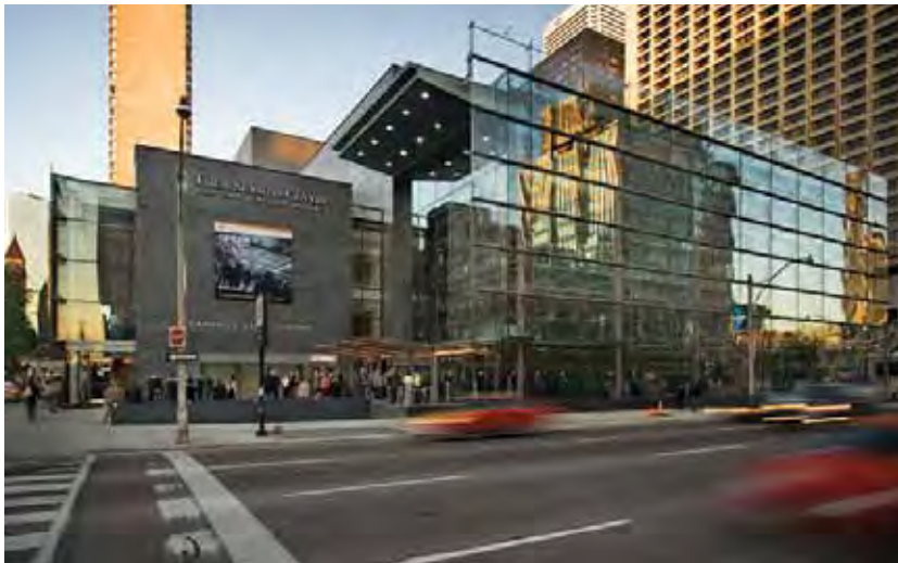
Four Seasons Centre for the Performing Arts. Diamond and Schmitt Architects. Photographer: Sam Javanrouh
