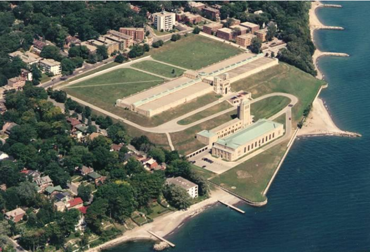
R.C. Harris Water Treatment Plant
