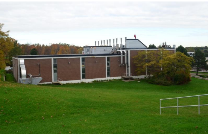
Highland Creek Wastewater Treatment Plant - Headhouse
