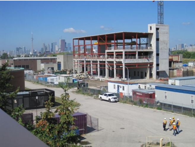
Ashbridges Bay Wastewater Treatment Plant – D Bldg .
