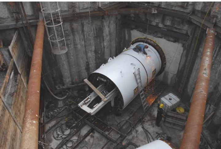
Entrance Shaft-Coxwell Sanitary Trunk Sewer Bypass
