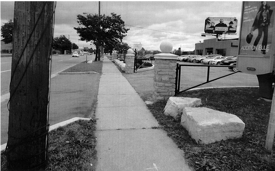
Photo # 2 - Showing 423 Evans Avenue and the posts and boulders
