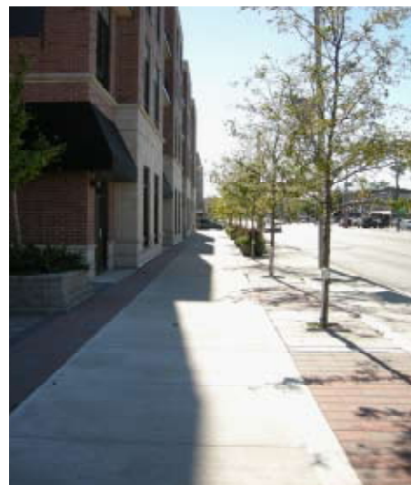
New streetscape on Dundas Street West
