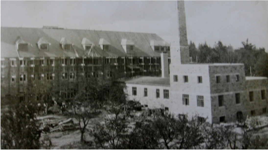
11. Archival Photograph, pre-1952 showing the north (service) wing (right) prior to the addition of the upper storey for the novitiate (Loretto Abbey Archives)
