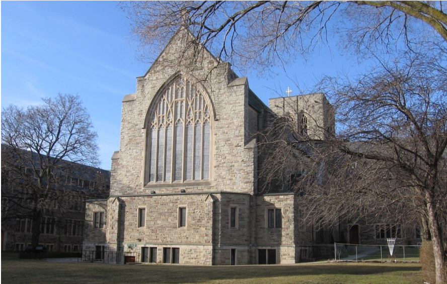
View of the rear (east) elevation, showing the Chapel that was completed in 1952 (June 2011)
