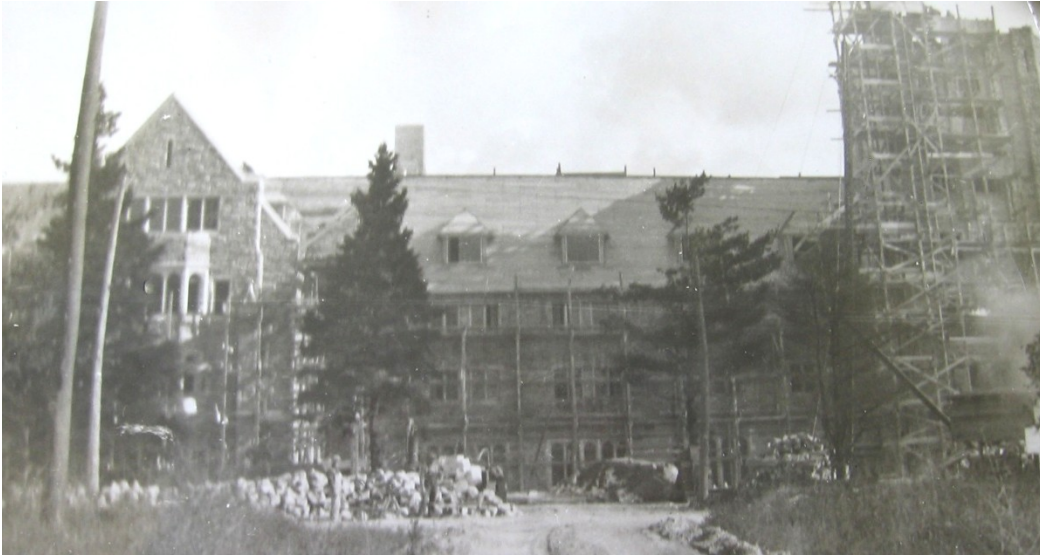
7. Archival Photograph, 1928 : showing the west wing with the tower (right) under construction (Loretto Abbey Archives)
