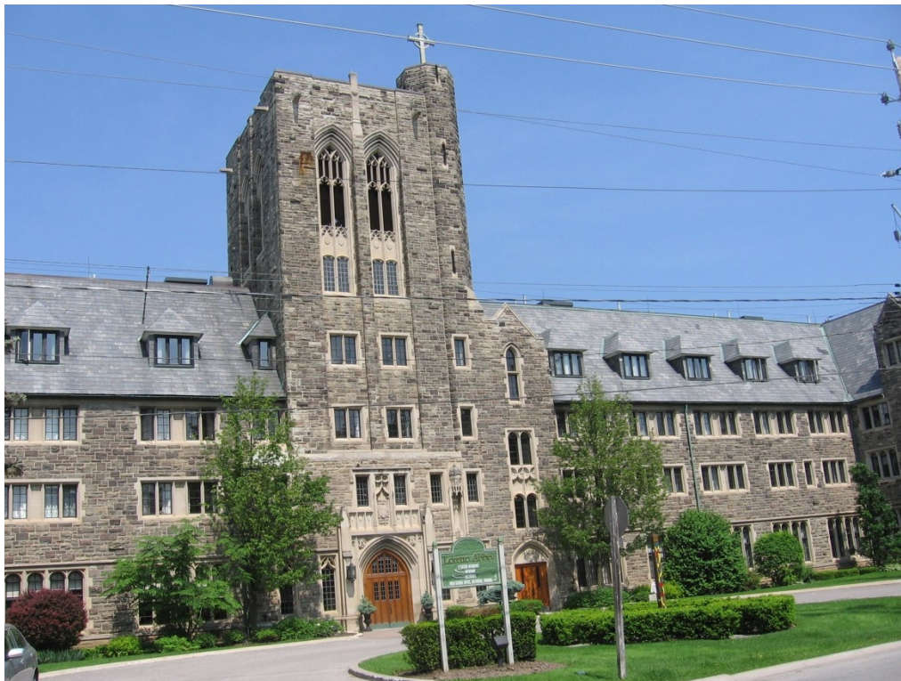
View showing the principal (west) façade and main entrance on Mason Boulevard (June 2011)
