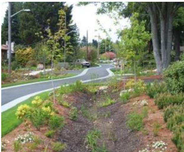
Typical Bioswale Construction Techniques
