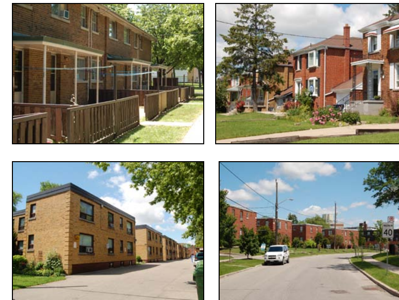
Figure 13: Existing Built Form
