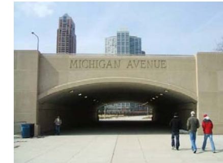
Wide, well-lit pedestrian underpass
