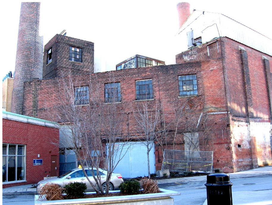
17. Photograph of the northeast elevation of the Hinde & Dauch Paper Company Power House with the two chimneys and the east tower (near the east chimney, left) rising above the rooflines of the complex (Heritage Preservation Services, February 2011)
