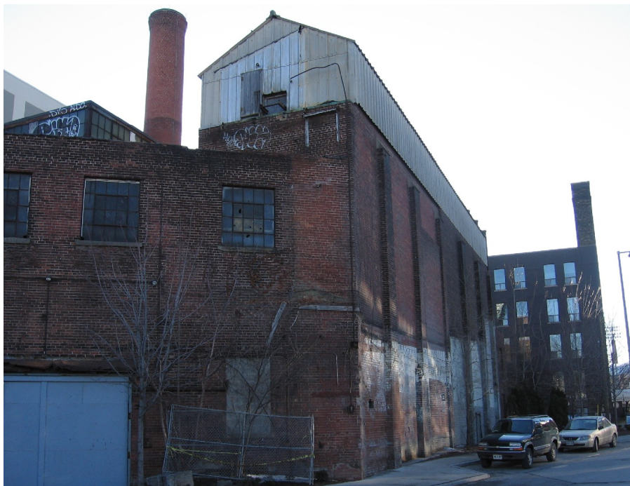
Photograph of the Hinde and Dauch Paper Company Power House, showing the north façade on Snooker Street (right) and the northeast elevation (left)
