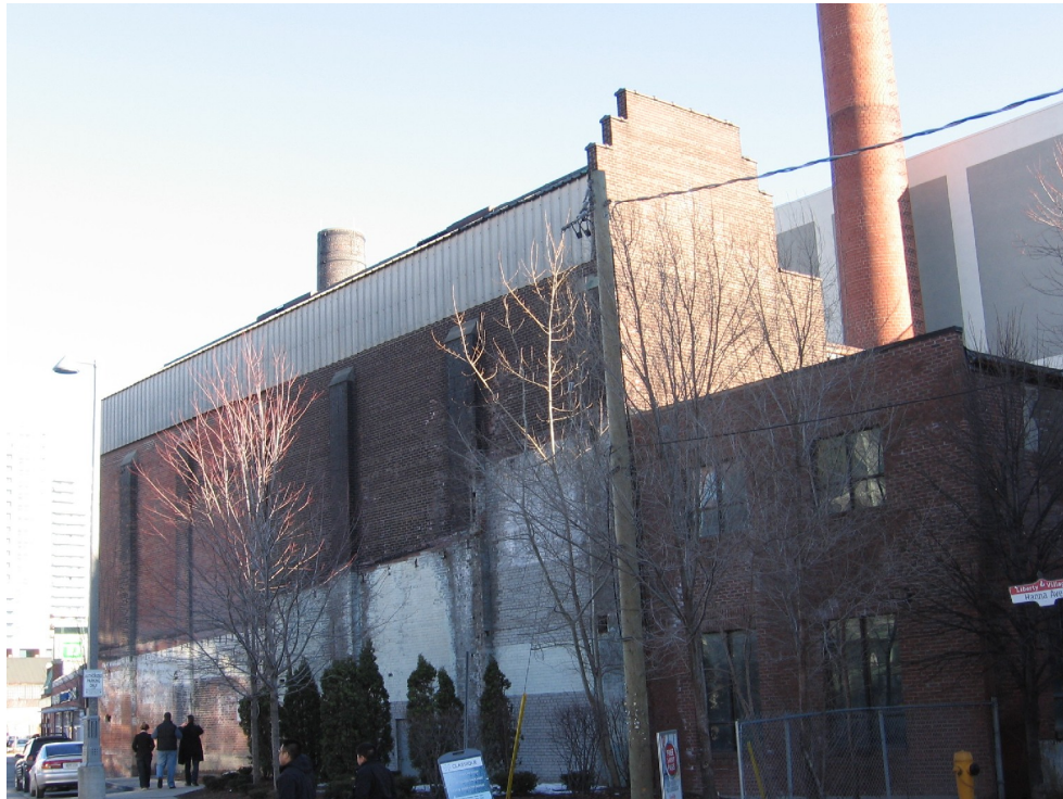
16. Photograph of the north elevation of the Hinde & Dauch Paper Company Power House (Heritage Preservation Services, February 2011)
