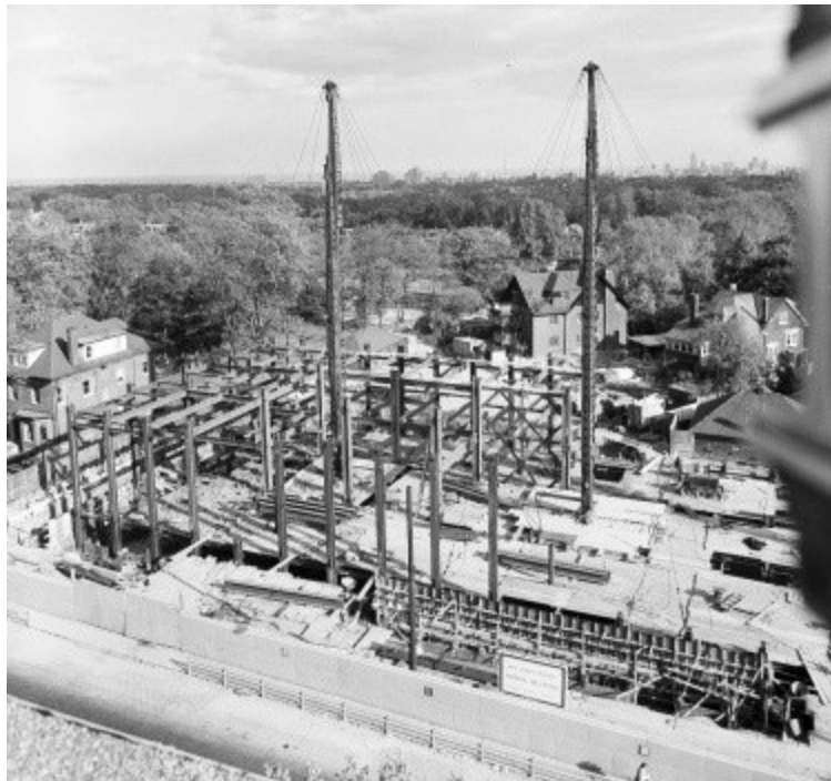
11. Archival Photograph, 1955 : showing the foundations for the Imperial Oil Building (Canadian Architectural Archives)
