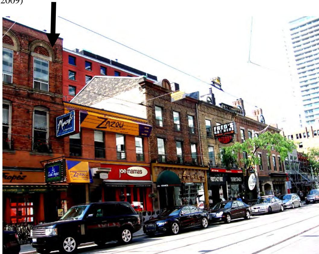
13. Photograph, King Street West, west of John Street ; showing the Joseph Devlin Building (left) (Heritage Preservation Services, 2011)
