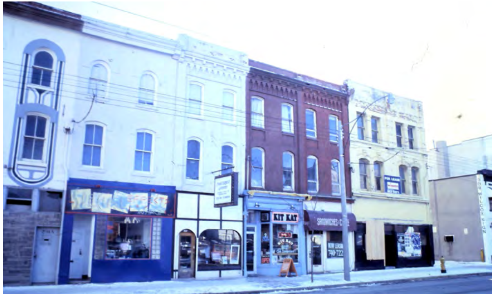
13. Photograph, 1991 : showing the James Devlin Buildings on the right, prior to the removal of the paint and the cornice detailing (Toronto Historical Board)
