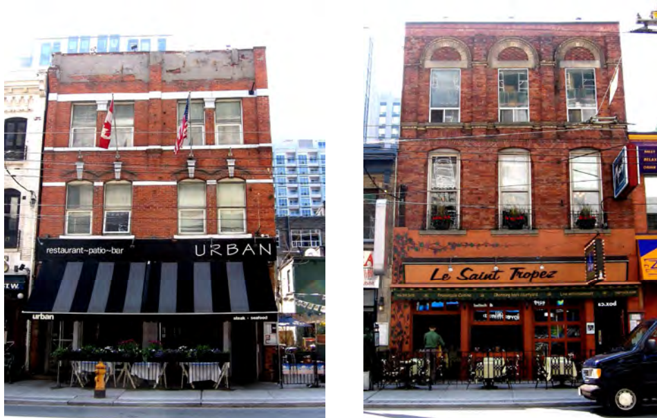
15. Photographs, 301 (left) and 315 (right) King Street West : showing additional late 19 th century commercial buildings in the same block as the subject properties. #301 was developed by Gardiner Boyd in 1886, following the construction of the subject buildings (Heritage Preservation Services, 2009)
