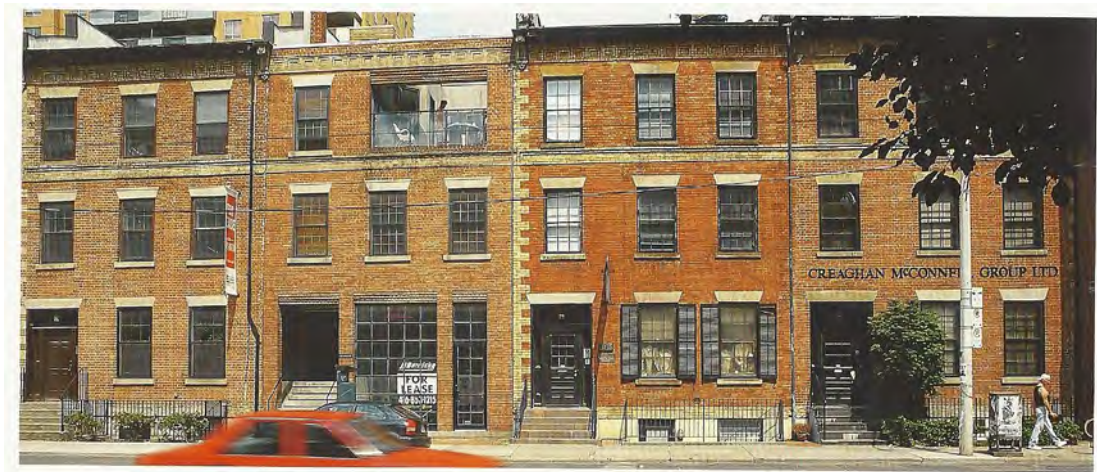
16. Photograph, Row Housing (1848), 191-197 Church Street ; showing the four-unit row housing that is attributed to John Tully and where #195 (second from the left) was replaced following a fire ( Old Toronto Houses , 42)
