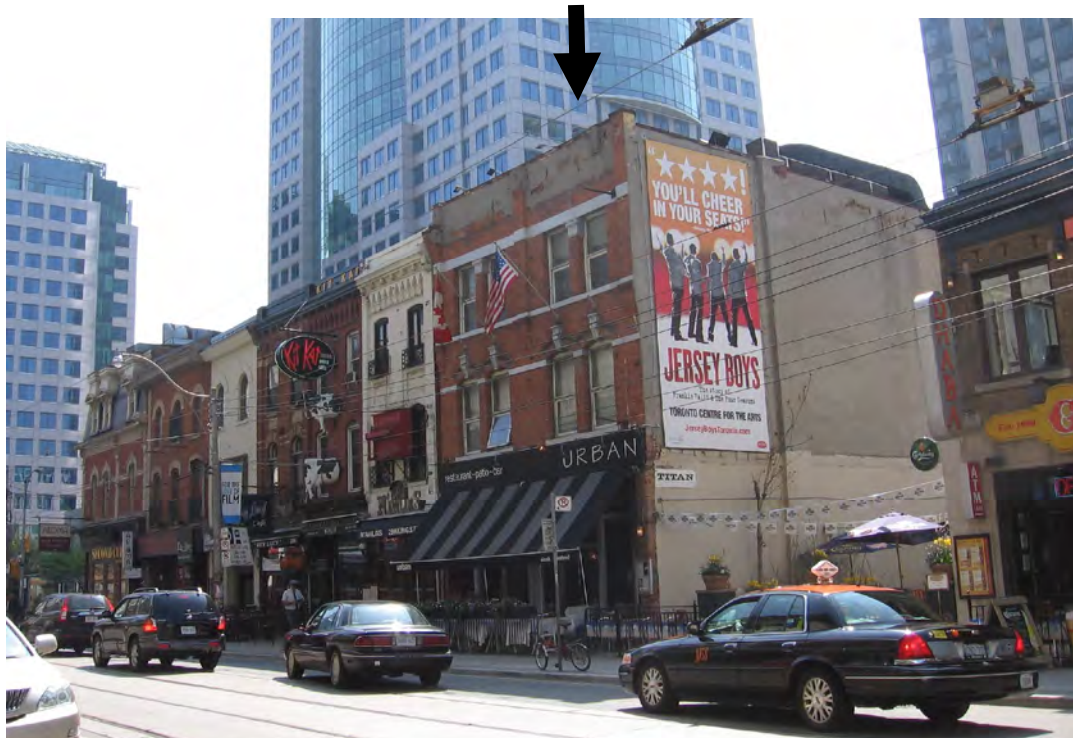
14. Photograph, 301 (303) King Street West : the empty lots to the west (right) originally contained three additional units developed by Gardiner Boyd in 1886 (Heritage Preservation Services, 2009)
