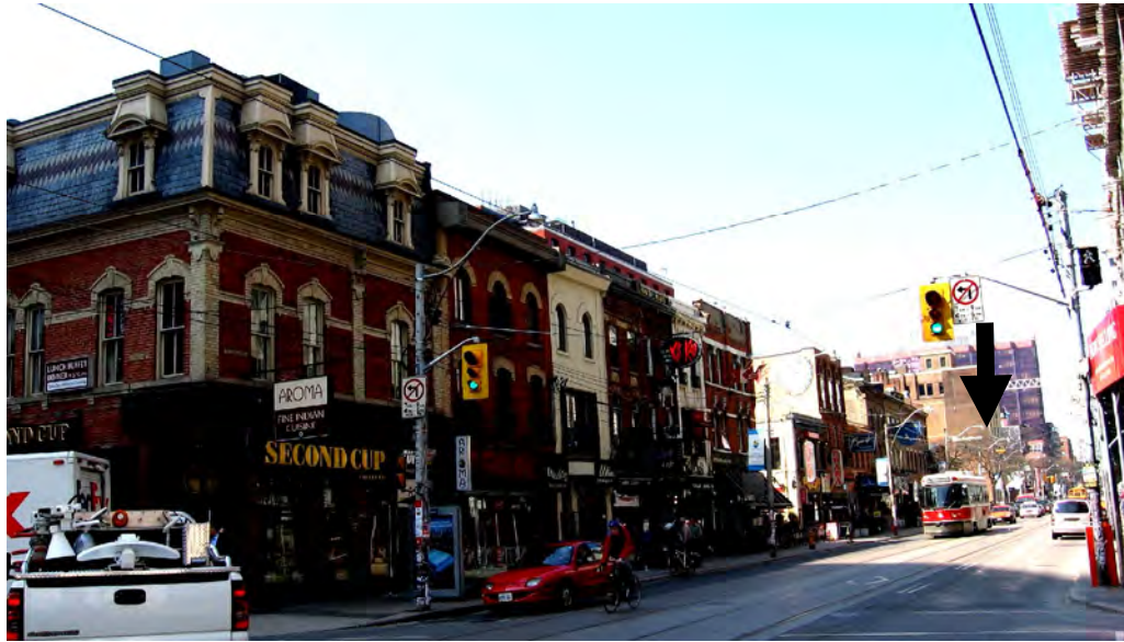
12. Photograph, King Street West, west of John Street ; with the arrow marking the location of the subject buildings in the block (Heritage Preservation Services, 2009)
