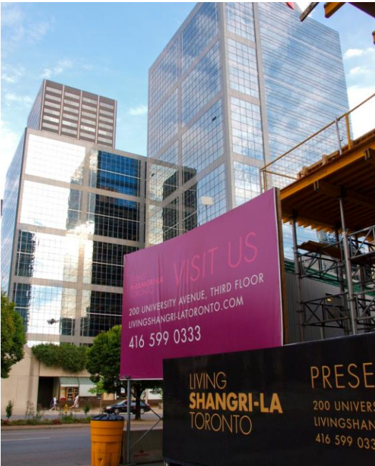
Figure 16 - Shangri-la development on University Avenue
