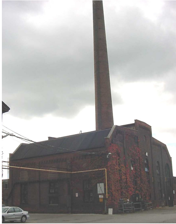
14. Photograph, Canada Foundry Company Powerhouse: prior to the demolition of the landmark smokestack in 2010 (Heritage Preservation Services)
