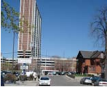
Before - view from South Station Street
