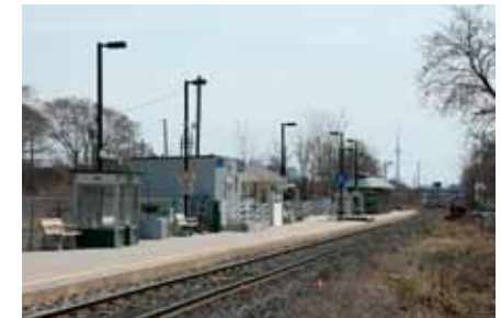
Existing GO station
