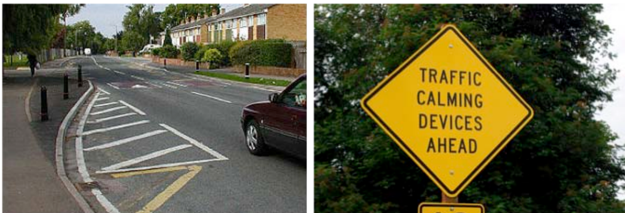
Figure 22: Traffic calming using curb extensions, pavement markings, speed bumps and signage Source: Wikipedia 2012 (left), stock.xchng 2007 (right)
