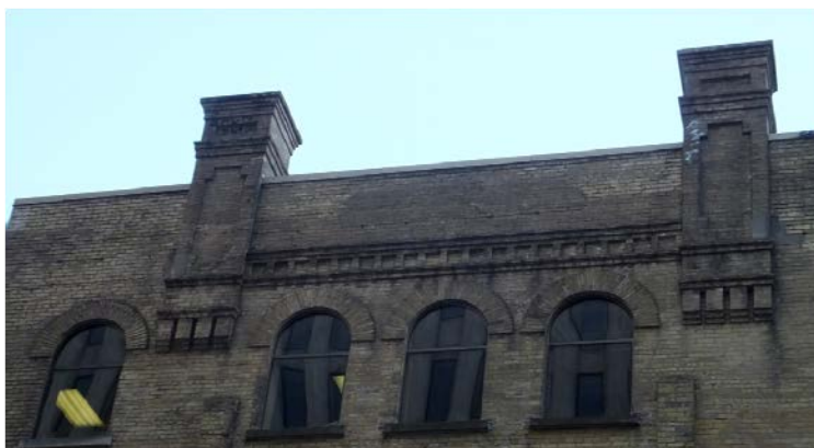
Above: detailing on south elevation Cover: Principal (east) façade on Yonge Street (right) & south elevation on Adelaide Street West (left) (Heritage Preservation Services, June 2012)
