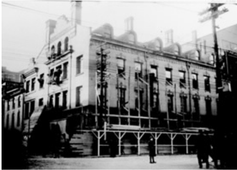
13. Archival Photograph, 1910: showing the Elgin Building prior to the alterations for Holt, Renfrew and Company. This view documents the mid 19 th century dormers and window detailing on the east façade (right), and the 1901 alterations to the south elevation (left) with the roof parapet and chimneys and the round-arched window openings (Toronto Reference Library, Item 4605)
