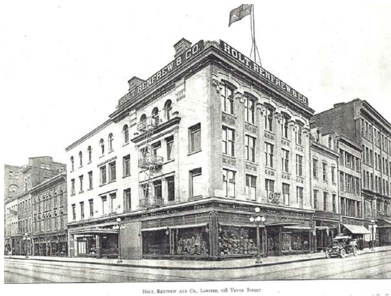
14. Archival Photograph, 1912: showing the building following the updating of the facades for Holt, Renfrew and Company with the extended cornice (later removed) and the retention of the chimneys and fenestration on the south elevation. A three-storey three-bay section of the Elgin Buildings with the dormers and window detailing remains to the north (right) and was later demolished ( Toronto, Canada's Queen City , unpagged)
