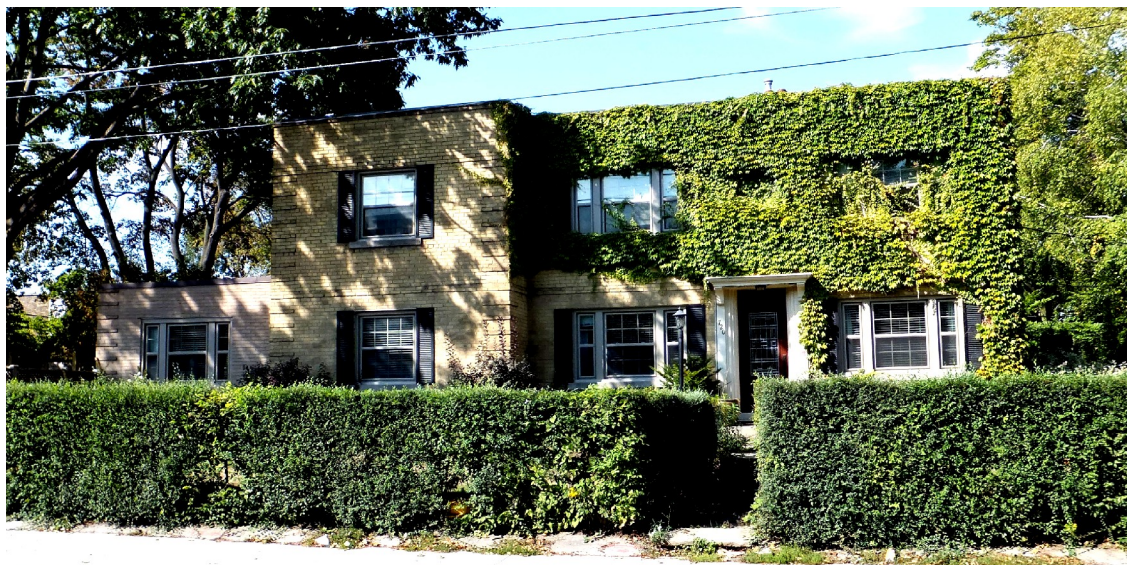
Above: south façade on Millwood Road Cover: south facade on Millwood Road (left) and east façade on Donegall Drive (right)
