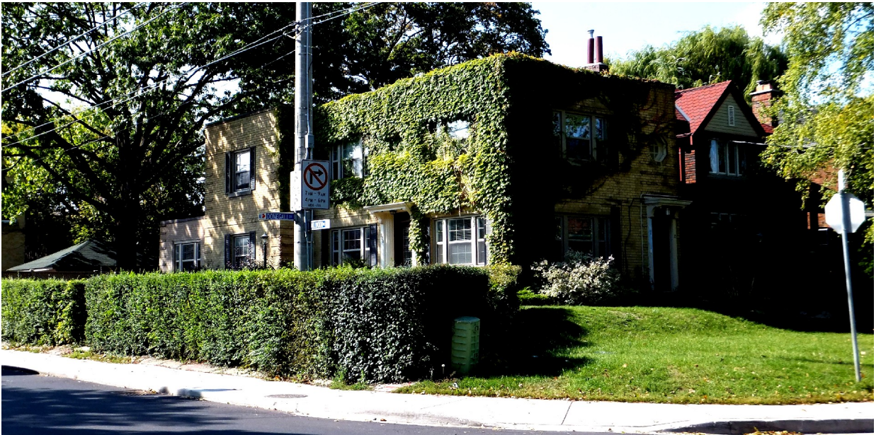
Above: south facade, 720 Millwood Road Below: south facade on Millwood Road (left) and east facade at 2 Donegall Drive (right)
