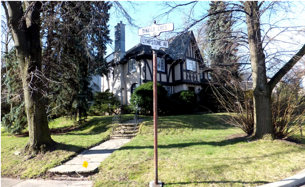
13. Photograph, 140 Dinnick Crescent : showing the Charles Langdon House on a corner lot near the southwest intersection of Dinnick Crescent and Lympstone Avenue (Heritage Preservation Services, April 2012)
