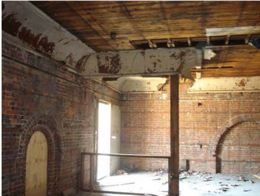
Remains of covered ceiling
