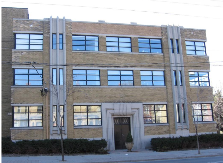
14. Charles Henson Laboratory, 833 King Street West : built in 1934, its design displays alternating bands of brickwork and fenestration and an entrance inset in a stone surround, but different decorative detailing than the Drug Trading Company's Administrative Office (Heritage Preservation Services, 2007)
