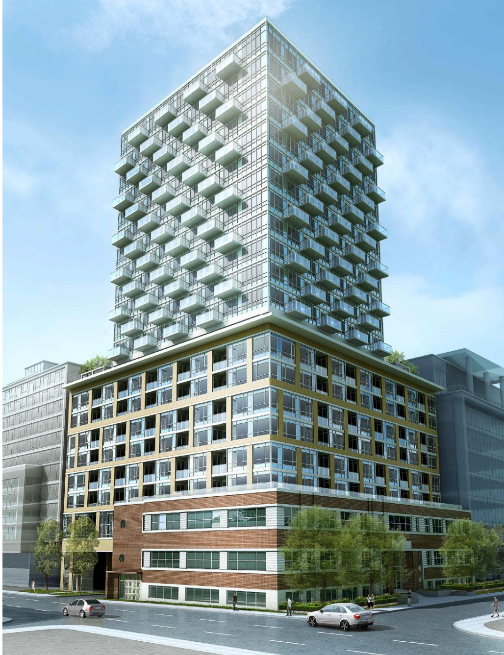
Rendering of the proposal for 25 Ontario Street showing the base building incorporating two elevations of the, Drug Trading Company Administrative Office, the middle tower component, and the upper tower component above.
