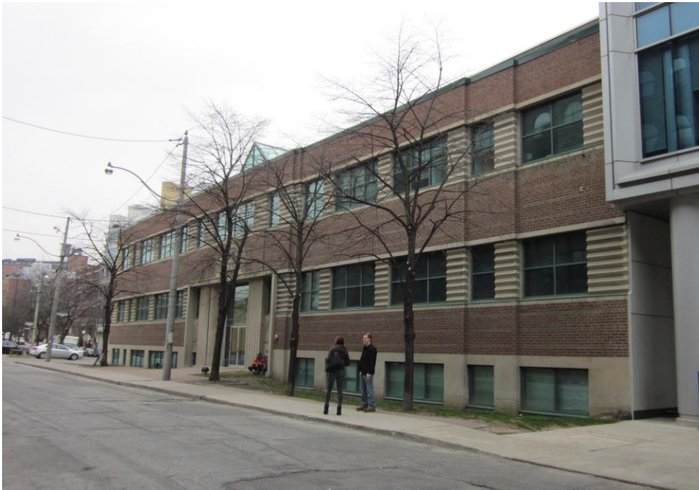
25 Ontario Street, Drug Trading Company Administrative Office, Ontario Street (West Elevation)
