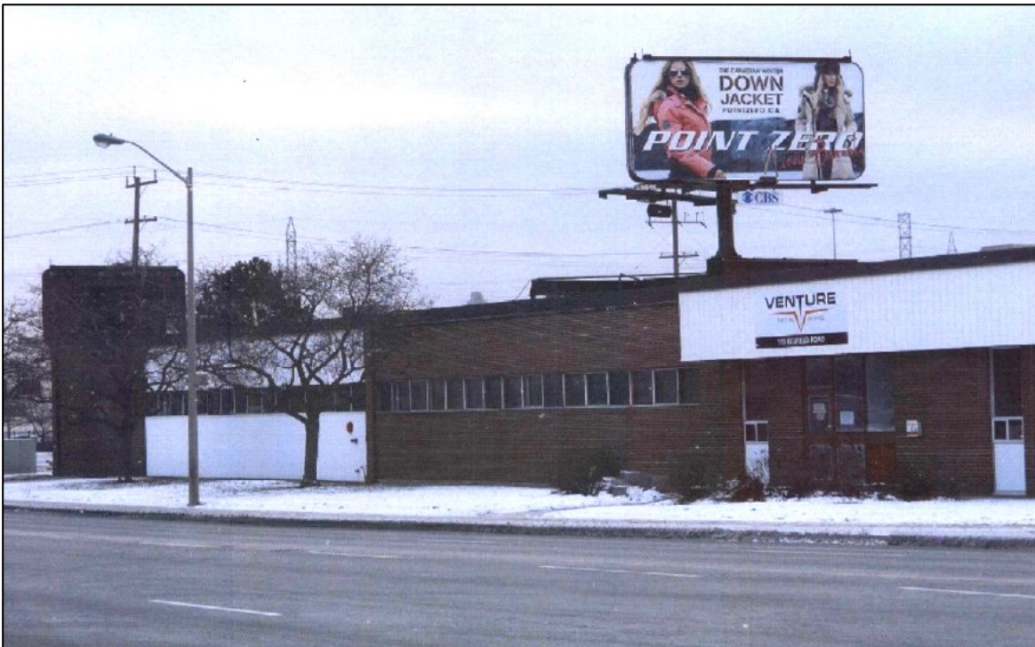
Figure 7 – Roof Sign proposed to be removed at 115 Belfield Road
