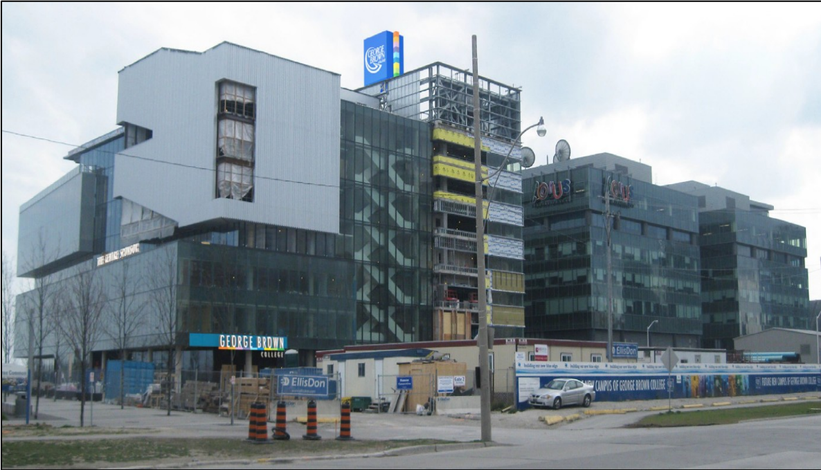
Figure 2: Rendering of north elevation of building showing the two proposed roof signs and one of the overhanging structure signs
