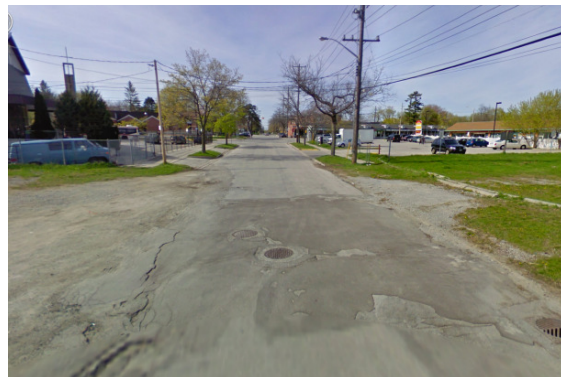
Streetscapes along the streets in the Village are in deteriorating conditions. Significant streetscape improvements are needed.
