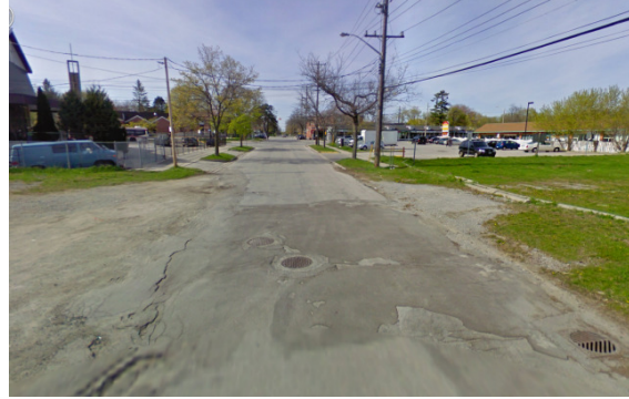
Morrish Road looking north
