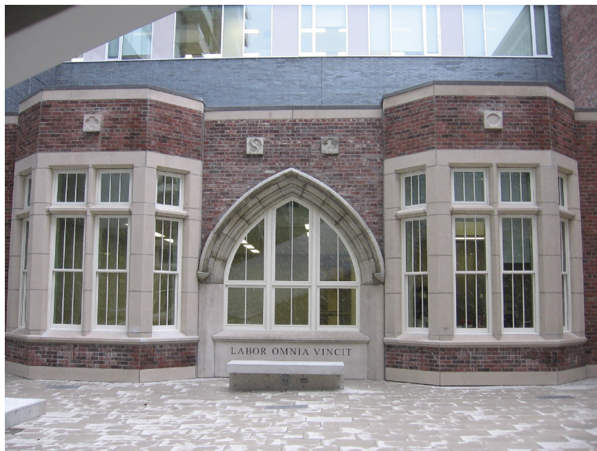
Photograph showing the south wall of the open courtyard on the interior of the new North Toronto Collegiate Institute where the first floor of the bay windows, the pointed-arch entrance opening, part of the brickwork, and the date stone "1912" (not shown) from the north wall of the original school have been incorporated (in the upper part of the wall, the four carved stones were taken from other parts of the school complex)
