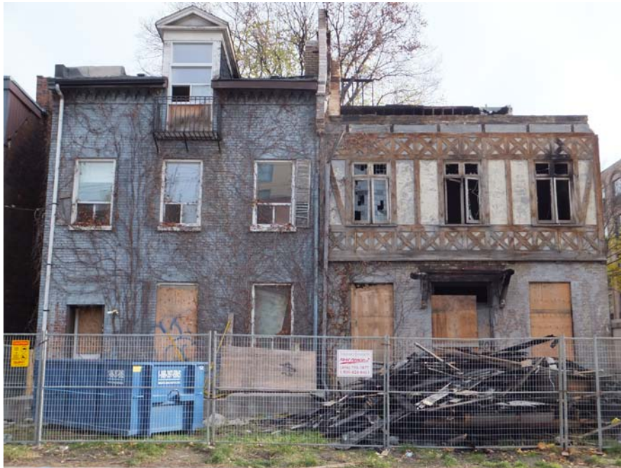
10. Photographs, 295 and 297 George Street, November 2011 : showing the principal west façades following the fire at #295 George in October 2011 (Heritage Preservation Services)
