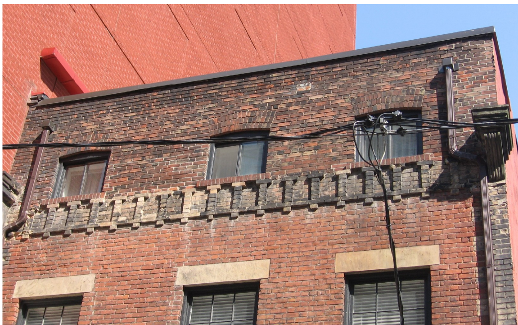
17. Photograph, 24 Mercer Street : showing the surviving roof detailing and the addition of the third storey (Heritage Preservation Services, 2011)
