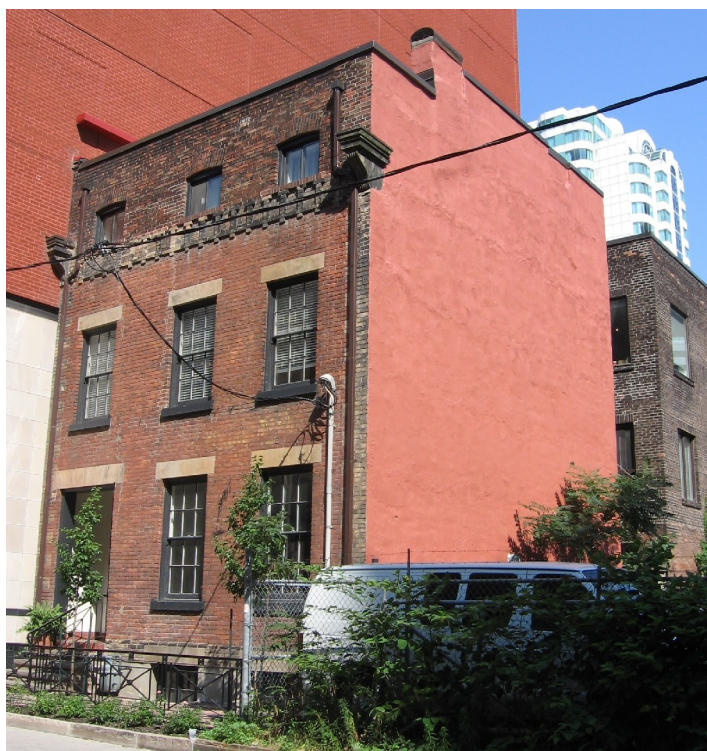
Above and cover: 24 Mercer Street showing the principal (south) façade, east wall and factory addition to the rear (north) (Heritage Preservation Services, 2011)
