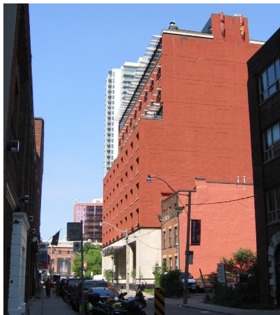
18. Photographs, 24 Mercer Street, 2011 : showing the south and east elevations with the factory extension (above) and the placement of the building on the north side of Mercer Street (below). (Heritage Preservation Services, 2011)
