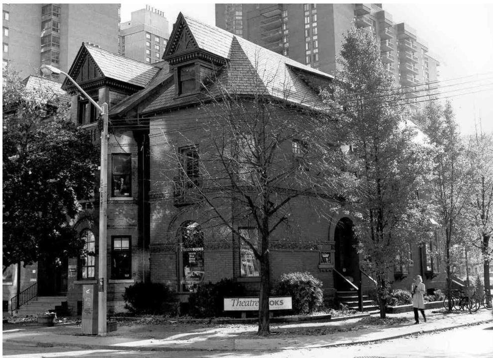
11 St Thomas Street - view of north and west elevations
