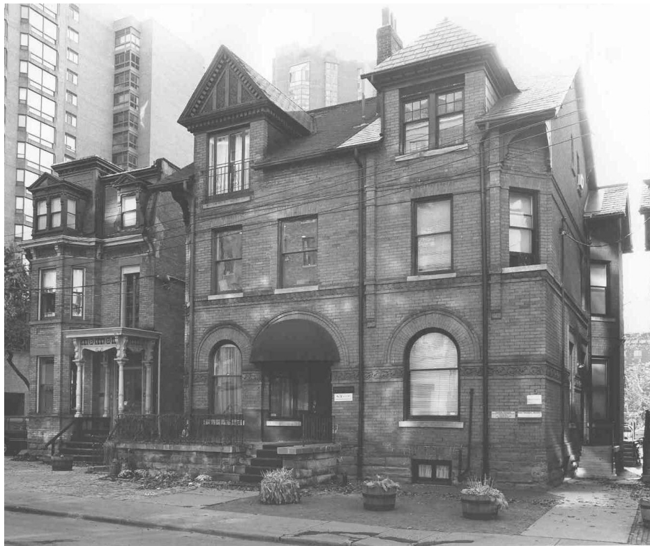
1, 3-5 Sultan Street – view of north (primary) elevation
