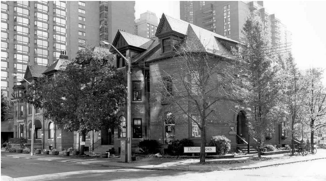
11 St Thomas Street and Sultan Street properties looking eastward
