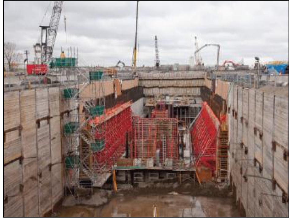
Toronto-York Spadina Subway Extension
