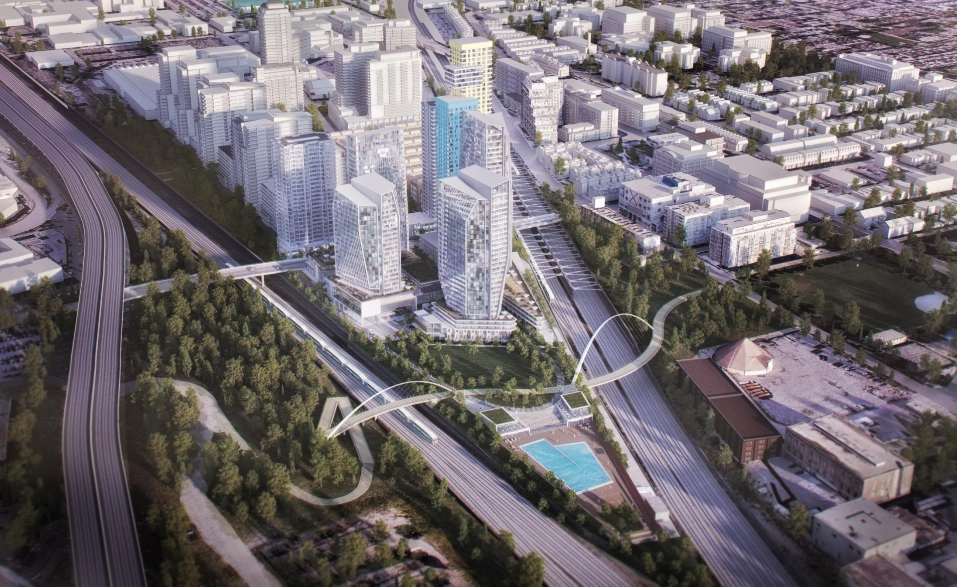
Looking NW across the Ordnance Lands & Strachan Ave Grade Separation towards Liberty Village
