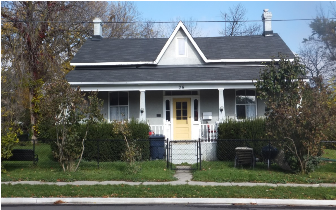
Principal (south) façade of the Richard Newborn House
