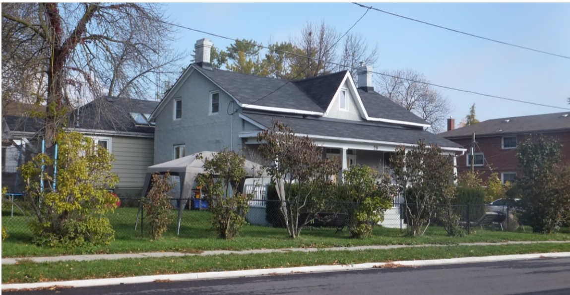
28 Daisy Avenue at the northeast corner of Twenty-Sixth Street in Long Branch
