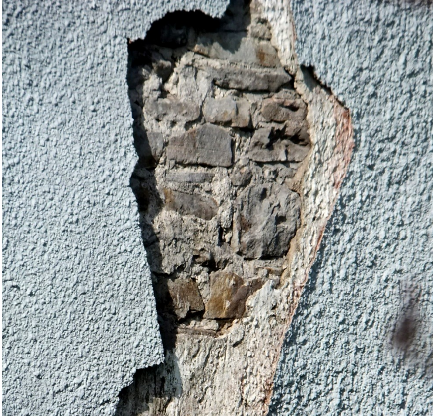
11. Current Photograph, 28 Daisy Avenue: showing the east elevation with part of the stonework exposed (Heritage Preservation Services, October 2012)
