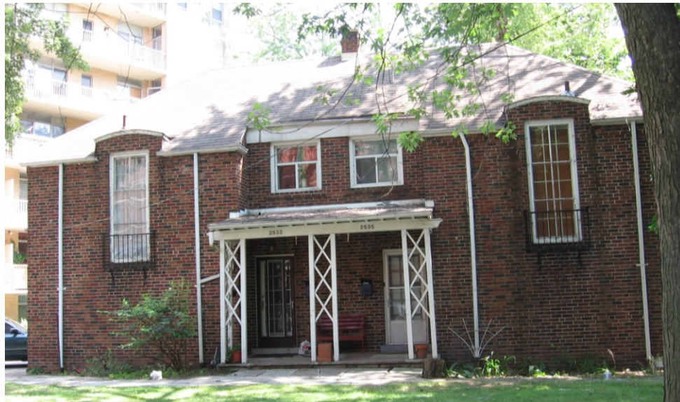
15. Photograph, 2533-2535 Lake Shore Boulevard West: showing the north facades of the semi-detached houses at the southwest corner of the estate that were built for staff accommodation (Heritage Preservation Services, 2010)
