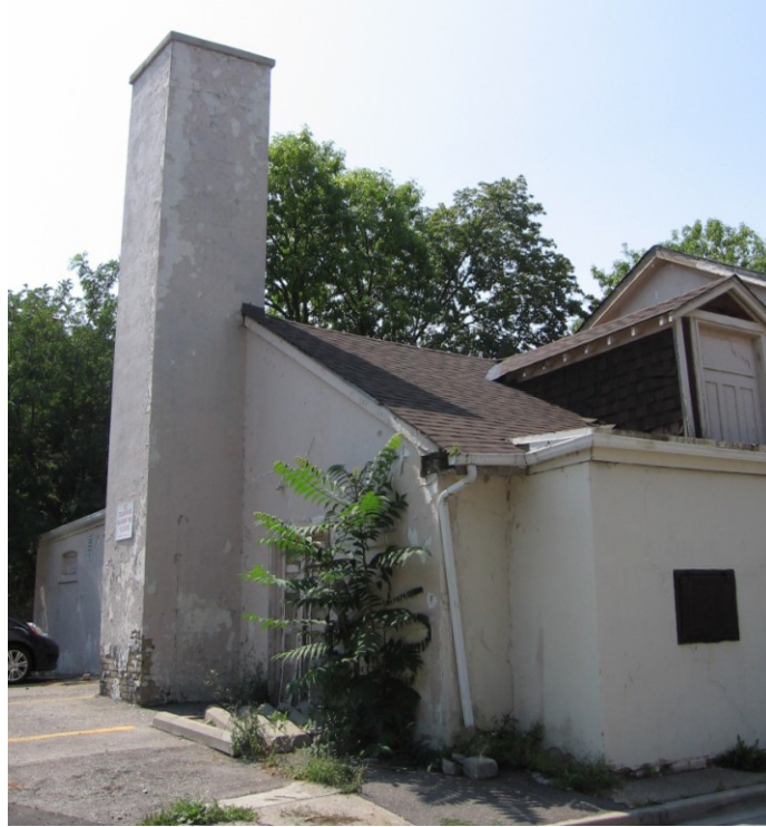
18. Photograph, 5 Douglas Boulevard: showing the power plant adjoining the housing at #7 and 9 Douglas (Heritage Preservation Services, 2010)
