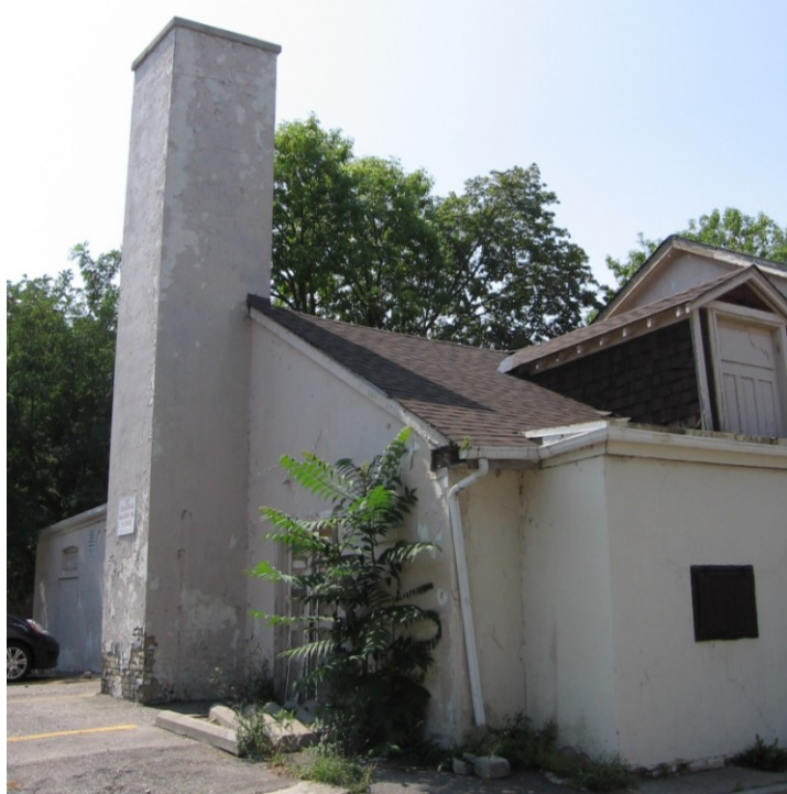
5 Douglas Boulevard : Power Plant – south end with the chimney (smokestack)
