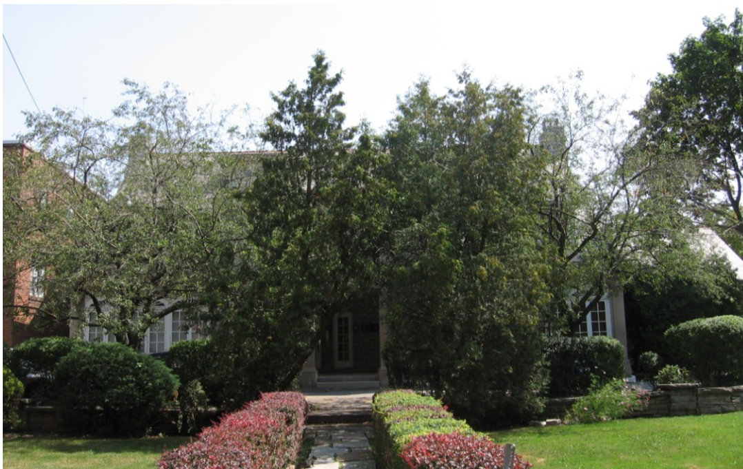
2523 Lake Shore Boulevard West: Ormscliffe, north façade
