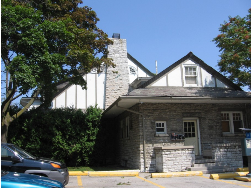
12. Photograph, 2523 Lake Shore Boulevard West : showing the west elevation of Ormscliffe, with the original south wing that is visible in the Construction magazine photographs in Image 5 (Heritage Preservation Services, 2010)
