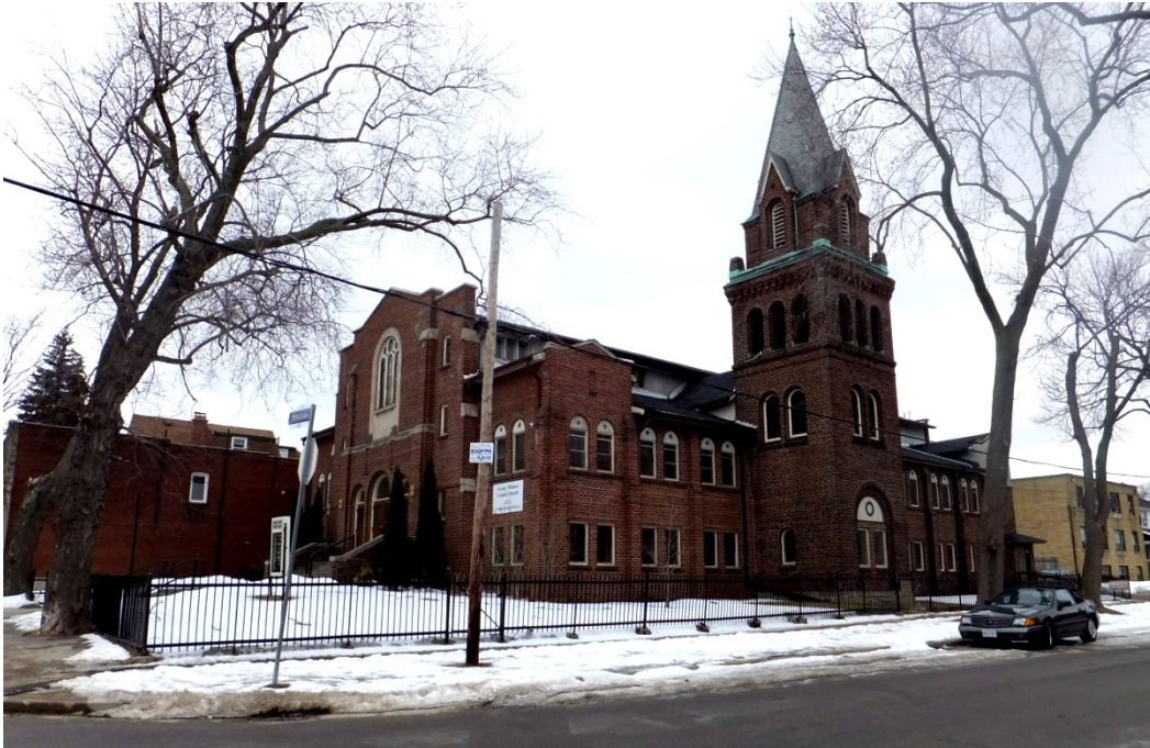
Principal (south) façade on Mimico Avenue (left) and south elevation on Station Road (right)
