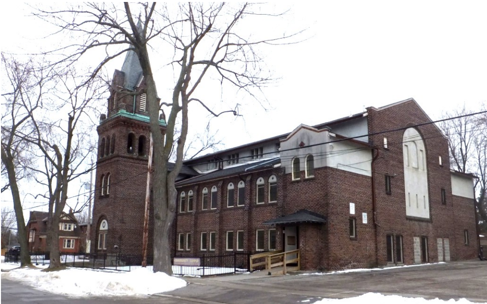
23. Current Photographs, 2 Station Road : showing the east elevation along Station Road, with the rear (north) wall (below right) (Heritage Preservation Services, February 2013)
