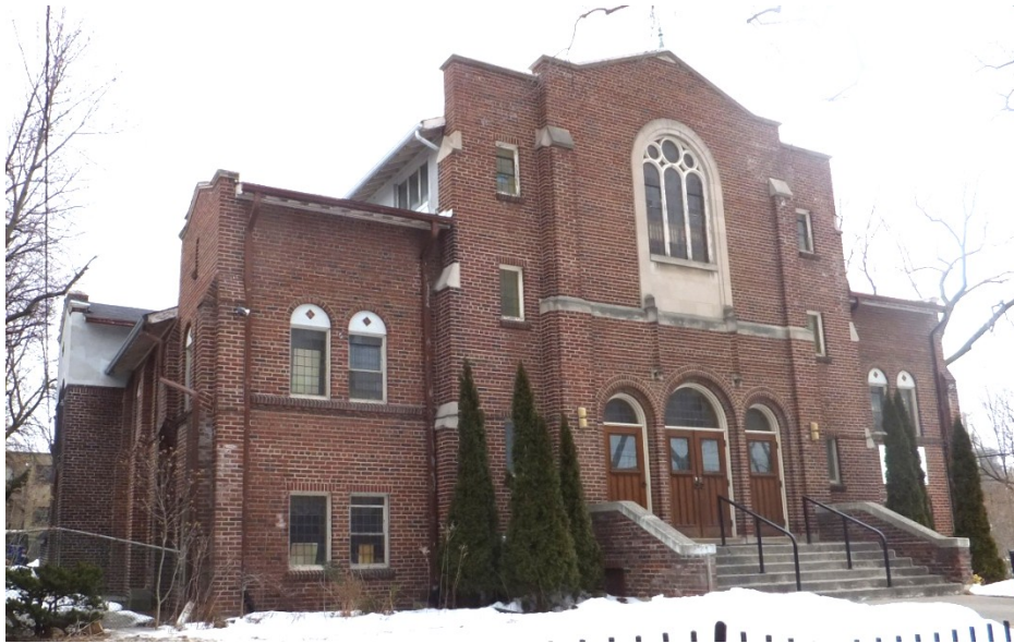
24. Photograph, 2 Station Road : showing the principal (south) façade on Mimico Avenue, with the west elevation on the left (Heritage Preservation Services, February 2013)
