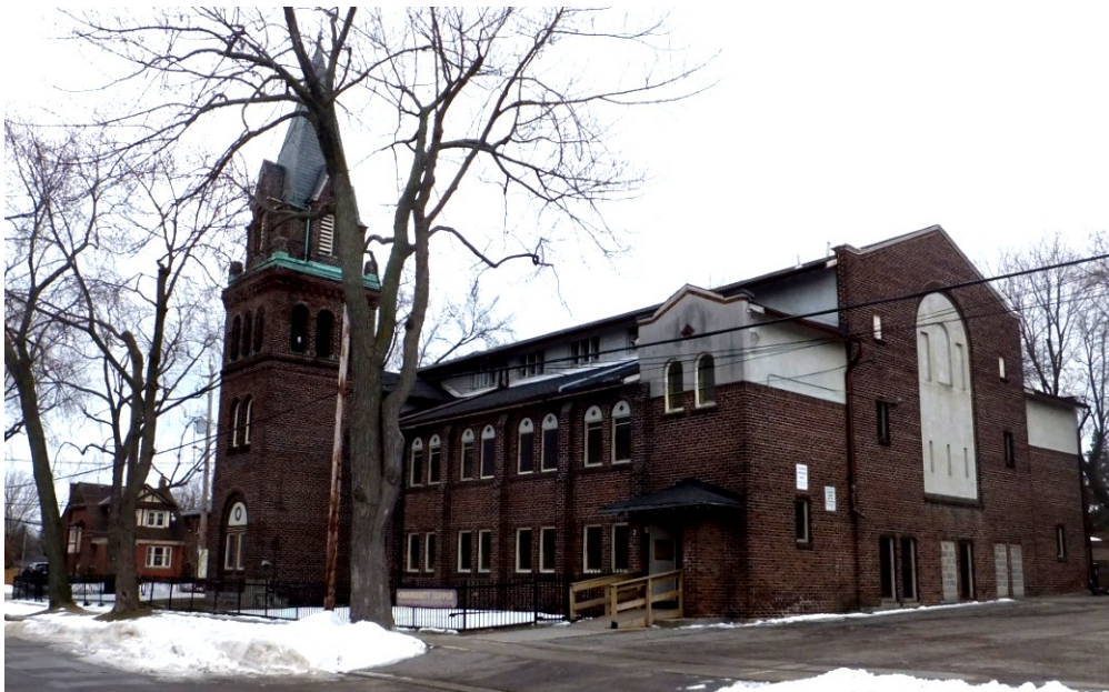
South elevation in Station Road (left) and rear north wall (right)
