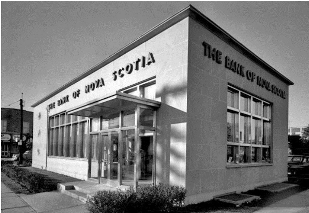
Archival photograph of the Mount Dennis Bank of Nova Scotia, the principal west facade and south elevation (photograph: 1952; CAA, Panda Associates Fonds, 52726-1, Unterman McPhail, p11)
