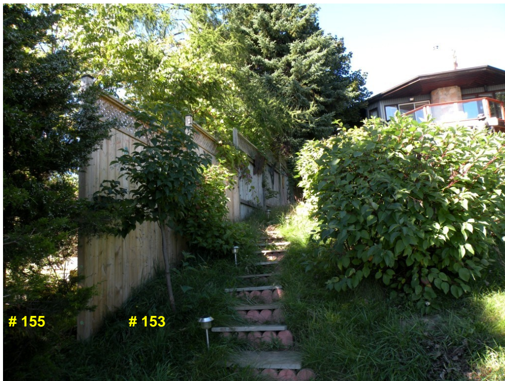
Attachment 5: Photos showing the section of the Fence in Question
