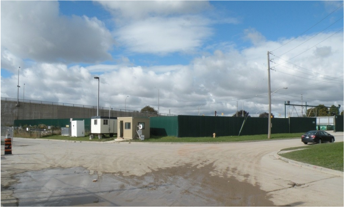
View from private street at rear and Etona Court flankage
