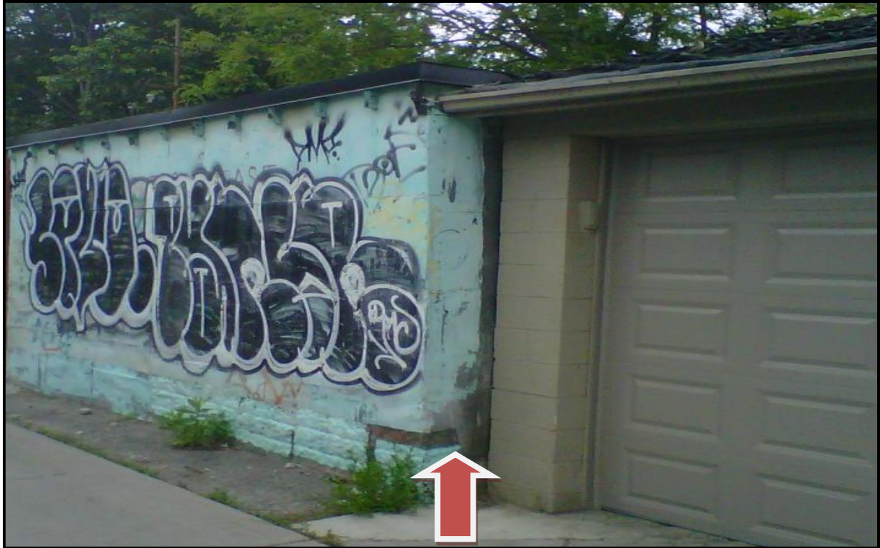
South Side of Garage at 182 Lisgar Street – Photo C taken June 18, 2013 by Christopher Pacheco
